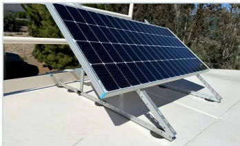
Roof-mounted module, welded reservoir — Pauma Valley CA
